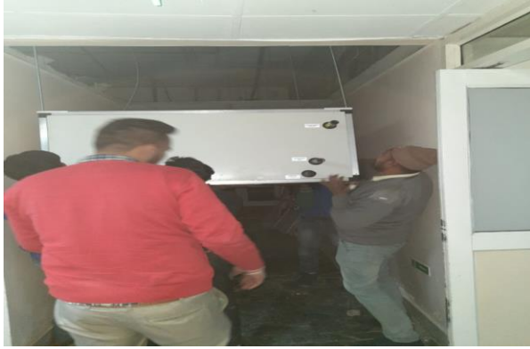
REPLACEMENT OF CONVENTIONAL AHU'S
